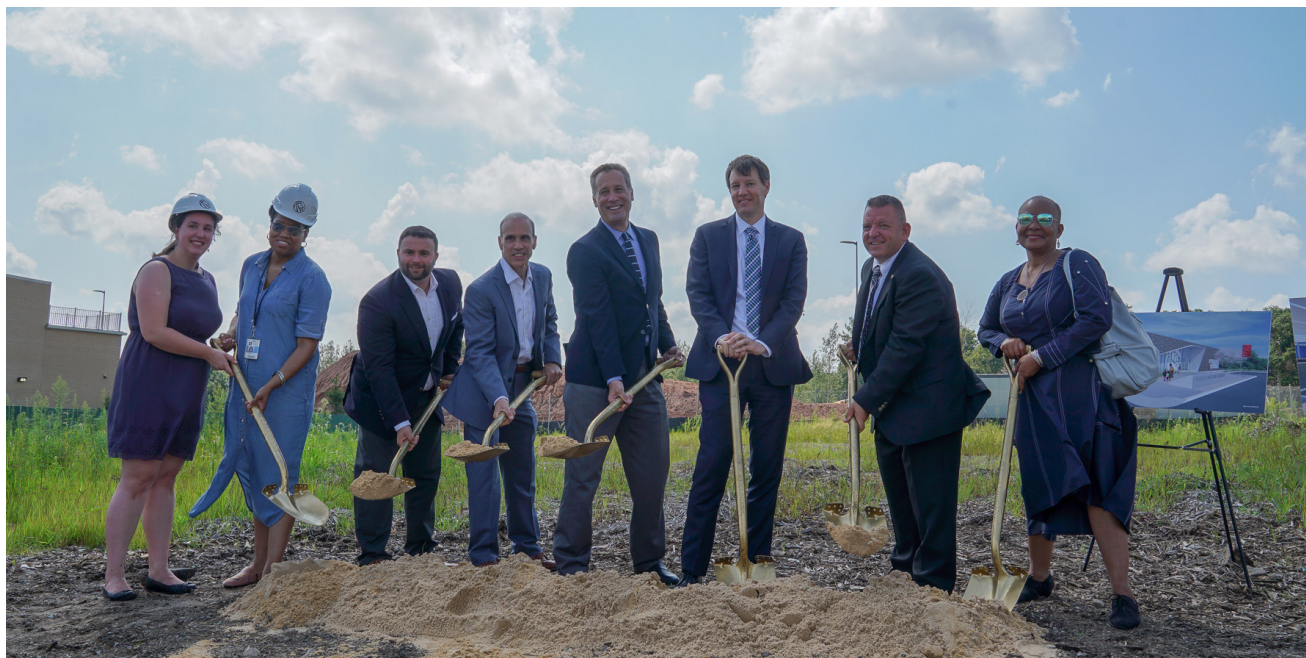
The Library, along with elected officials and community members, kicked off construction of the new Charleston Library on Staten Island with a ceremony at the site of the new branch, slated to open in 2021.
